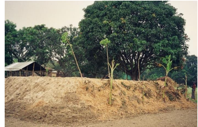
Photo 3.3 Planting vegetation on the periphery of raised mound
