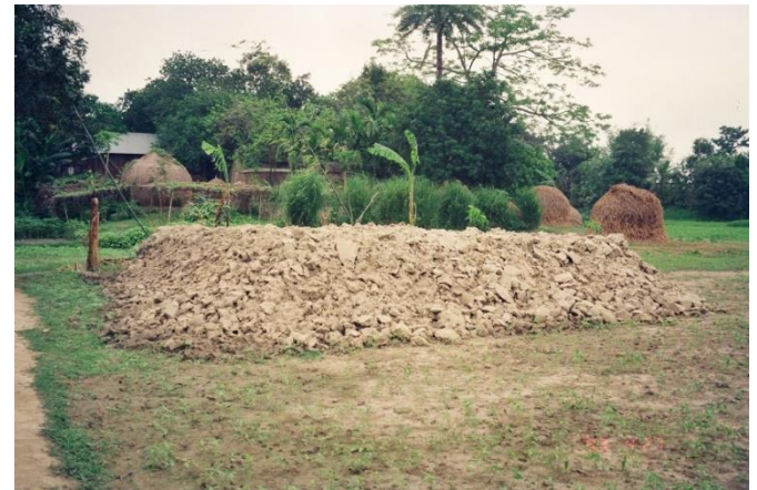
Photo 3.2 The raised mound on which huts will be built
