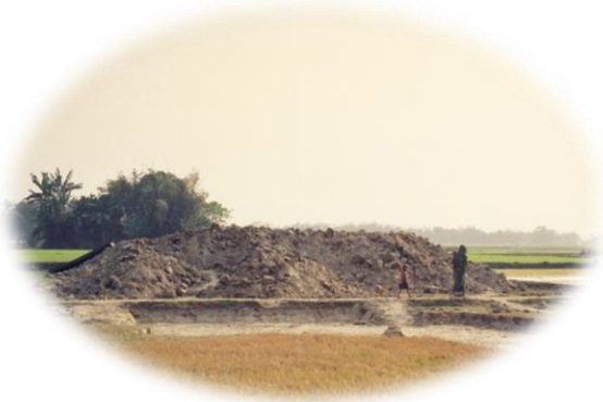
Construction of raised mound by digging soil
