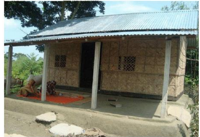
Photo 3.4 Earthen plinth consisted of clay soil
