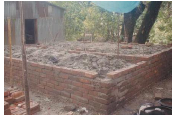
Photo 3.5 Brick perimeter wall plinth filled with soil
