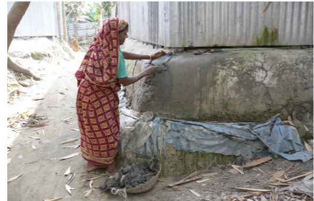
Photo 4.2: Plastering of plinth with muddy soil mixture
