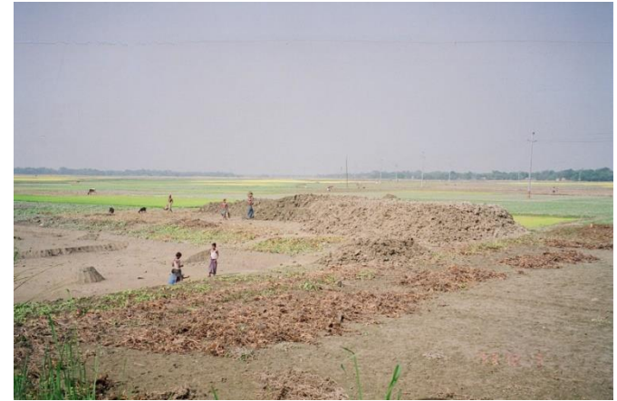
Photo 3.1 Digging of soil for raised mound
