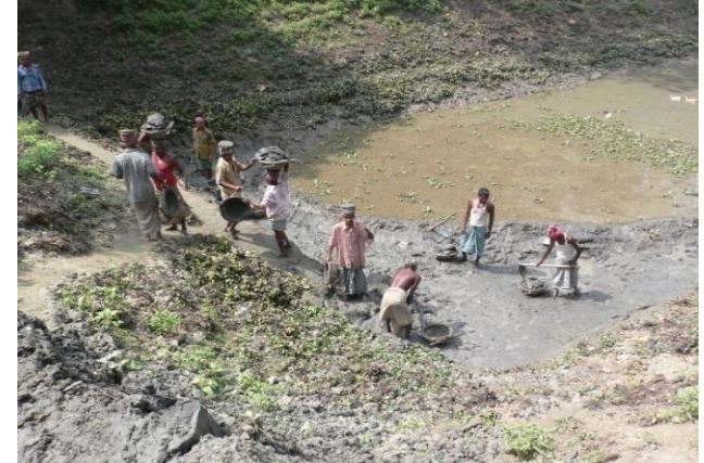
Photo 4.1: digging of clay/muddy soil to the homestead
